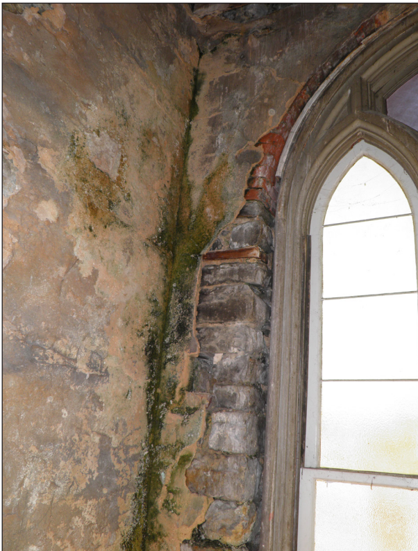
Disrepair inside the South Tower.
