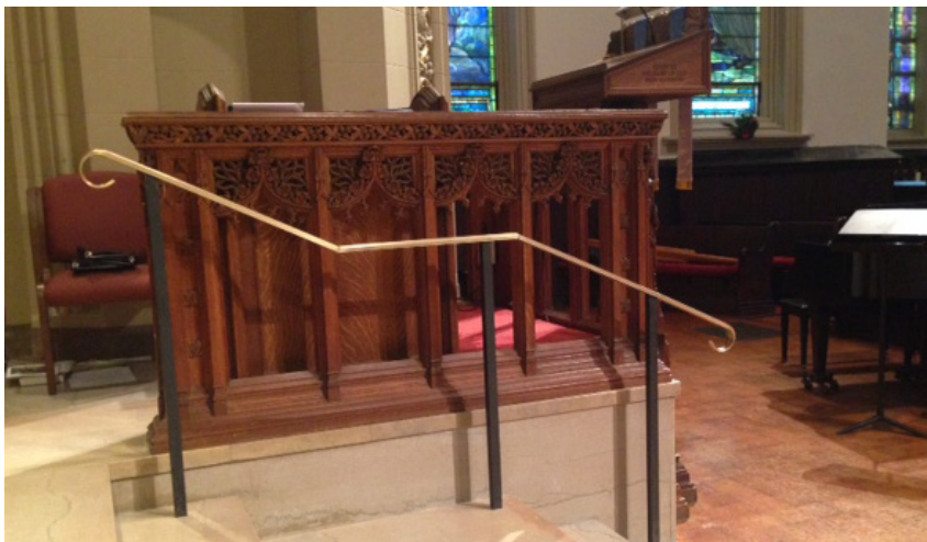
The first fruits of the Capital Fund were installed in December—new Chancel stair rails will improve safety and accessibility within the Sanctuary.
