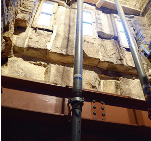
On Jan. 1, construction crews spent five hours installing the horizontal steel beam pictured here to secure the internal structure of the South Tower.
