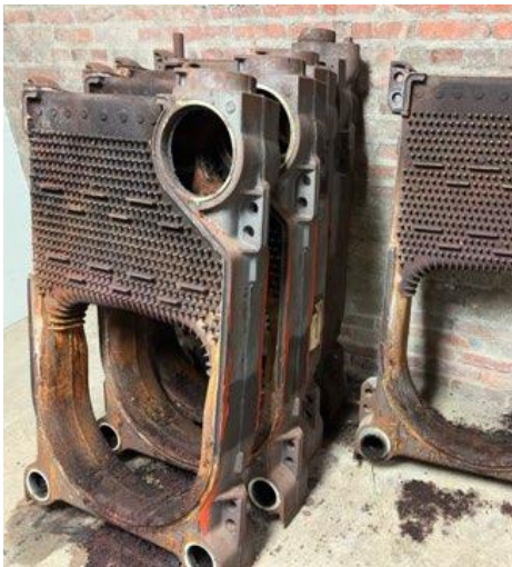
THE OLD BOILER HAD TO BE REMOVED IN PIECES
