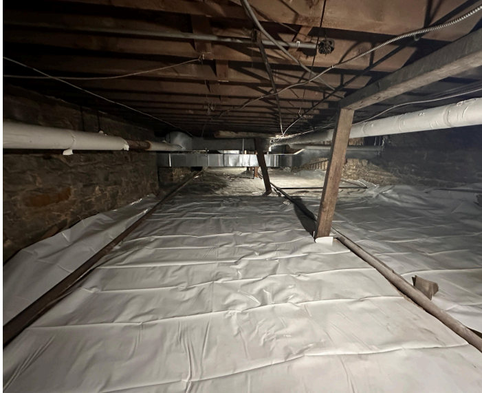
Crawl space under the Sanctuary after abatement.
